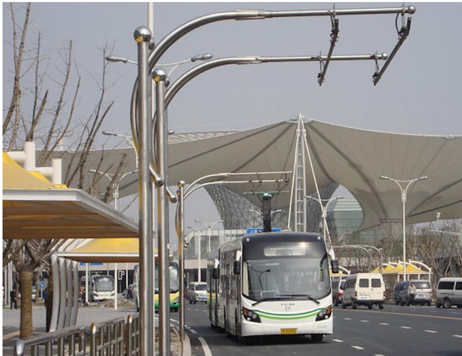
Figure 3.7: Trolleybus Charging Point at Bus Stop, Shanghai
